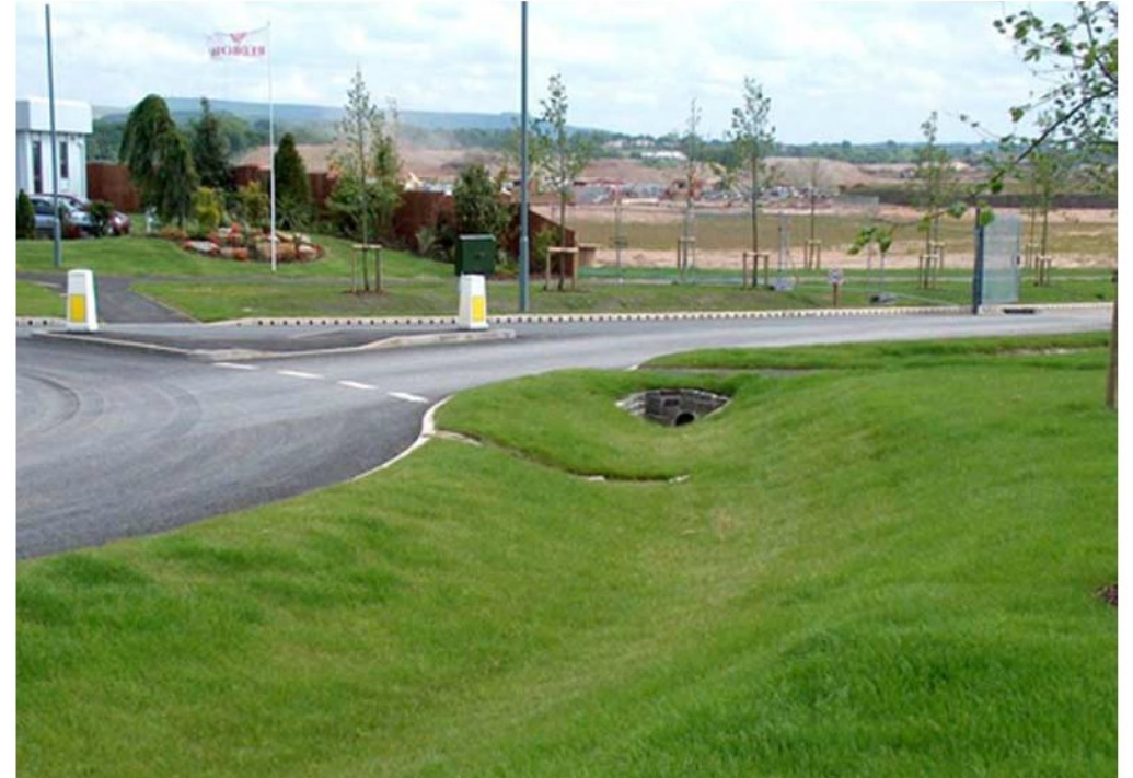
Figure 1: Sustainable urban drainage system
